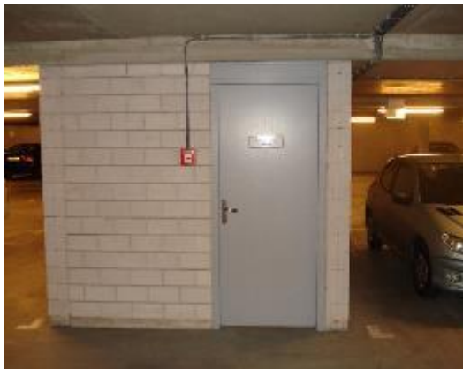
Emergency exit in the underground car park
