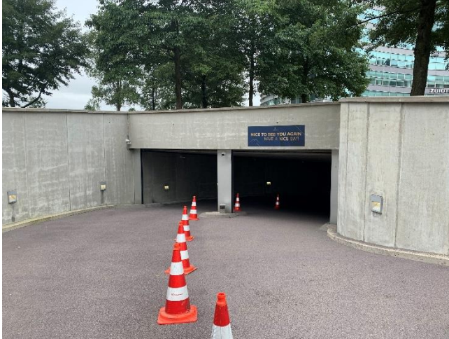
Entrance underground car park
